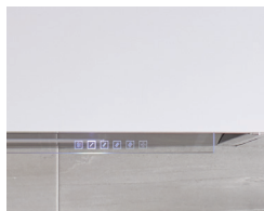
Hood mounts inside custom cabinetry; only the control panel shows.
